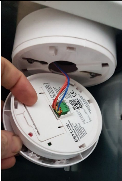
FIGURE 7: BATTERY REPLACEMENT
